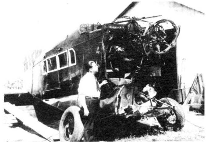
No. 4 airplane, NC132H, crashed in Milwaukee Harbor on takeoff in a tailwind. It was piloted by Jim Benedict. Here Doerflinger examines the remains.
