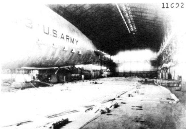
The ex-Navy Blimp, Army's D-3, moved aside in the hangar at Langley Fd. for floor inspection of the ROMA envelope before erection. (Photo-USAF #11692)
