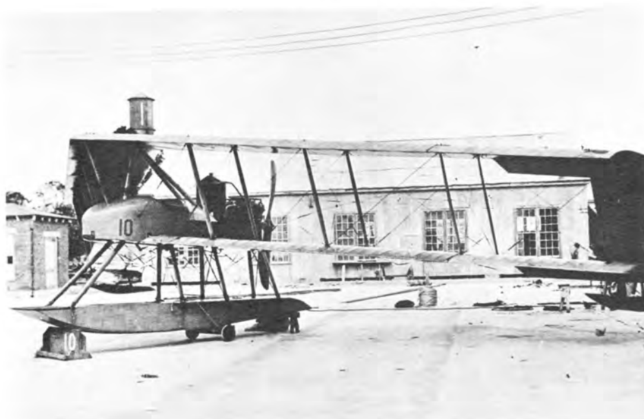
Another view of the AH-10, taken in November 1916. On this aircraft, Starling Burgess eliminated the "bustle" and gave the wings uniform camber. (National Archives 80-G-180221)
