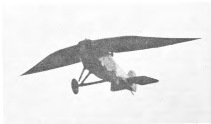
In 1921 the "Tin-side red-devil" (Martinsyde Semi-Quaver) was converted from a biplane to a monoplane by the installation of an "Alula" wing. Mr. Reginald W. Kenworthy was test pilot. The strange wing design was of great inspiration to B. D. Thomas (Flight)
