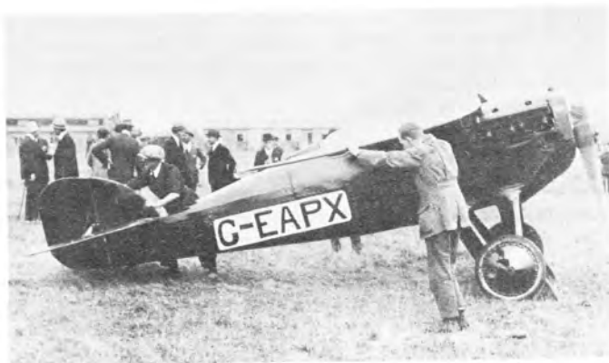
In 1921 the "Tin-side red-devil" (Martinsyde Semi-Quaver) was converted from a biplane to a monoplane by the installation of an "Alula" wing. Mr. Reginald W. Kenworthy was test pilot. The strange wing design was of great inspiration to B. D. Thomas (Flight)
