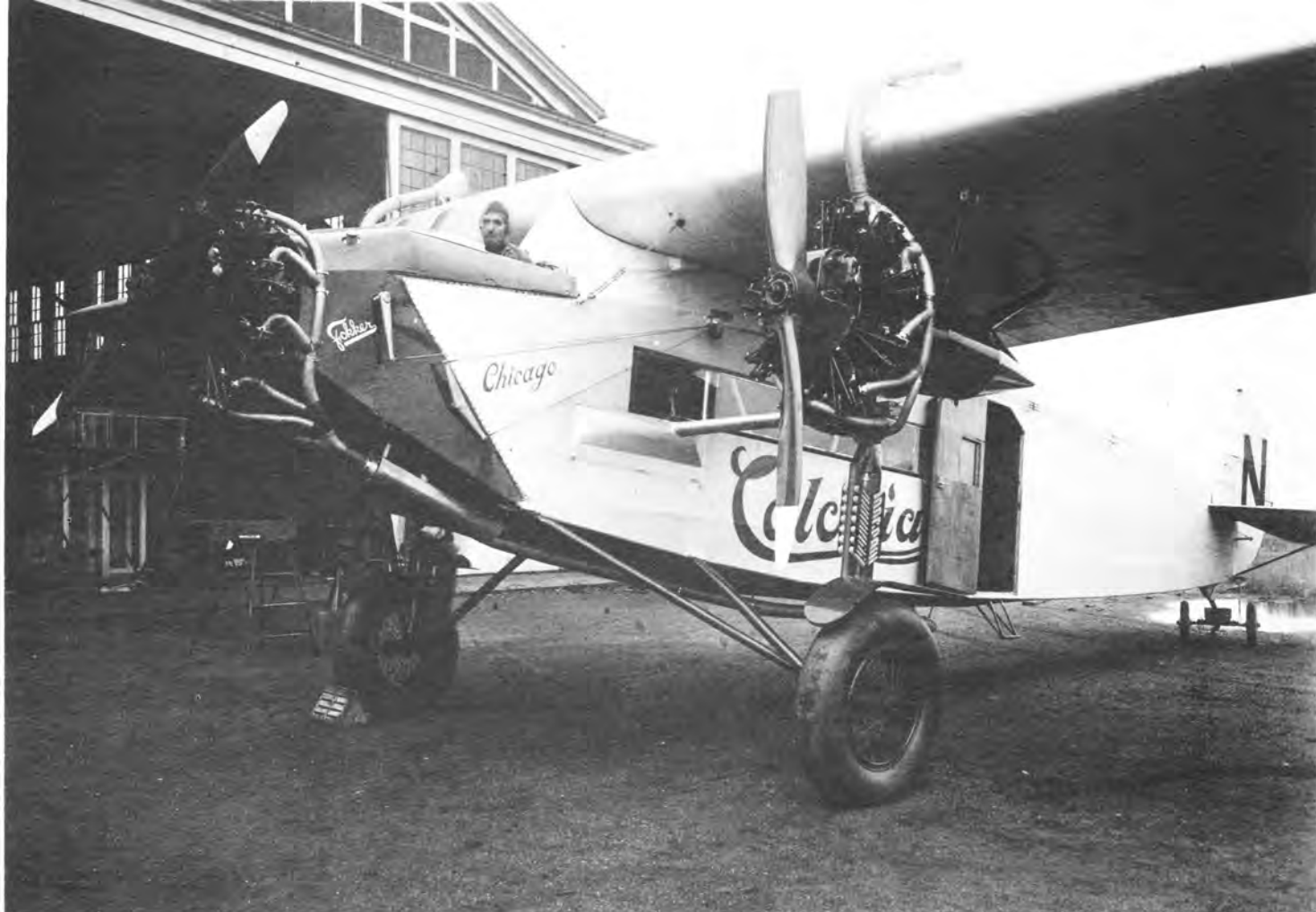
The first Fokker C-2 in original form with open cockpits and Wright J-4 engines. Enclosure was soon added, but distinctive arrangement of metal panels on nose was retained for all C-2/RA-1 through -3 models. (American Fokker 419)
