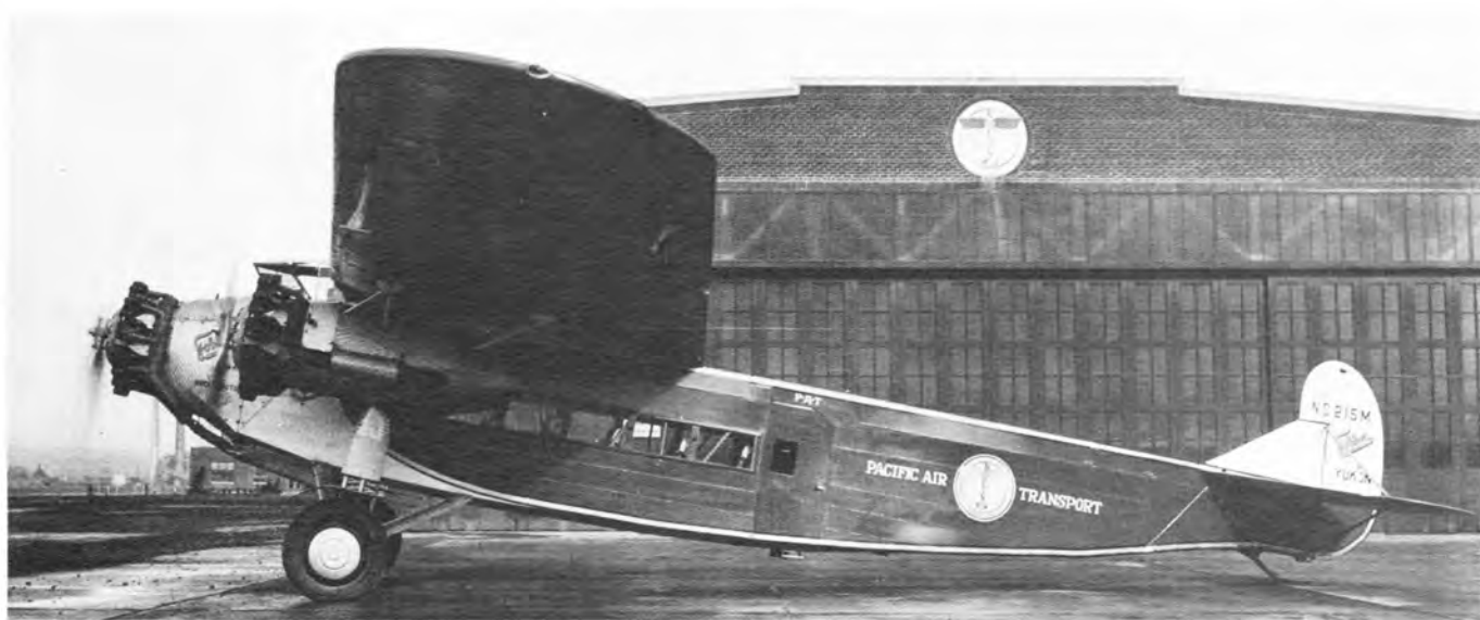
F-10A, NC-215M, C/N 1044, in Western Air Express colors, was used by West Coast Air Transport and Pacific Air Transport before flying for WAE. Lower longeron reflexed for use of a steerable tail wheel but tail skid retained. (Boeing 4421)
