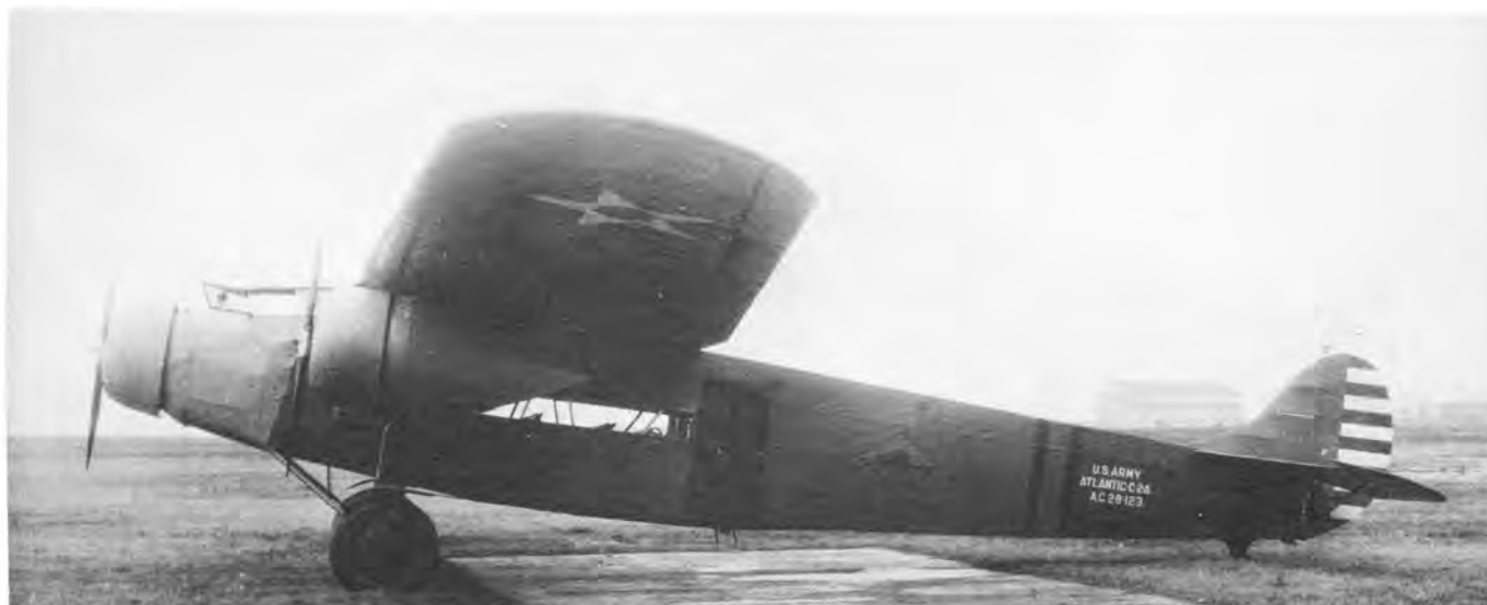
The fifth Fokker C-2A, 28-123, on loan to N.A.C.A. at Langley Field, Virginia for tests of the N.A.C.A. engine cowlings, which were under development at the time. (N.A.C.A. 3285)
