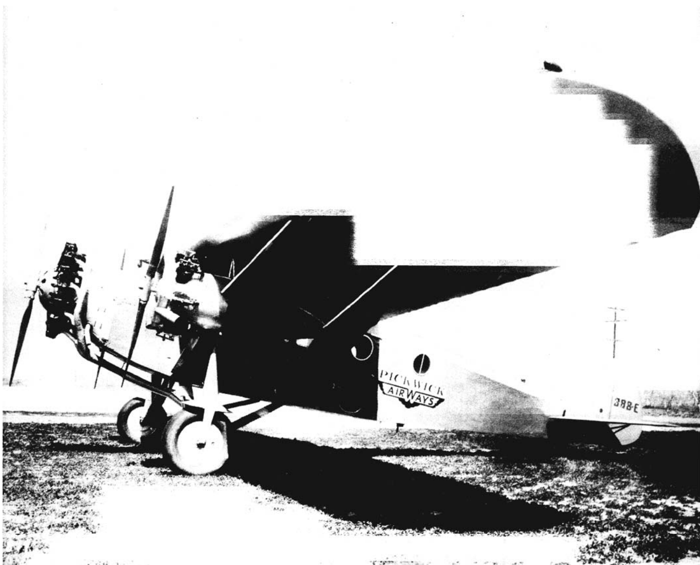
One of Pickwick Airway's Bach 3-CT-6 eight passenger transports during first months of operations. The Bach was powered by a single Pratt & Whitney Hornet engine and two, smaller Comet engines giving a total of 835 hp. At a weight of 8000 pounds, normal cruising speed was 125 mph. (M. L. Bailey)
