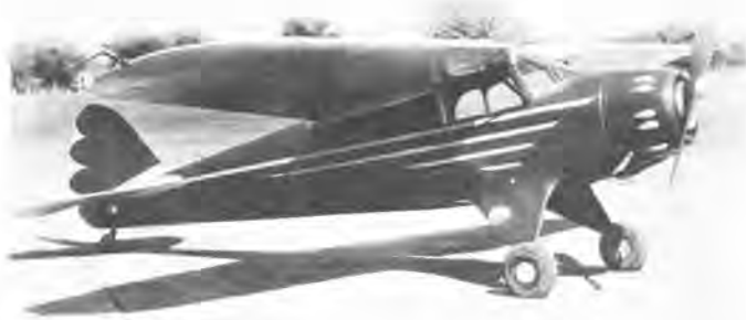
Fahlin SF-1 built in 1934 and powered by 85 hp Pobjoy "R" radial. Registration X271Y. (John Underwood)
