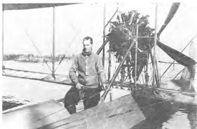
Frank Coffyn in Burgess Model I Flying Boat with its 20 cylinder Anzani engine. (Smithsonian A-41,479-a)
