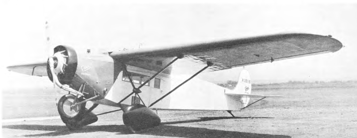
Special 300 hp J-6 Universal with open cockpit and anti-noseover wheel built for George Graves of New York. A J-5 Universal, 1548, C/N 420, was also fitted with the extra wheel for TELA Railroad Co. Honduras. (Fokker Photo 1771)
