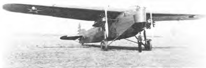
American Fokker Model No. 5, the Army XLB-2, as originally delivered in 1927 with P & W "Wasp" engines and forward-slanted V-windshield. Windshield was later expanded to a complete enclosure similar to later Army C-2s and commercial F-10s. (Wright Field Photo 33326)
