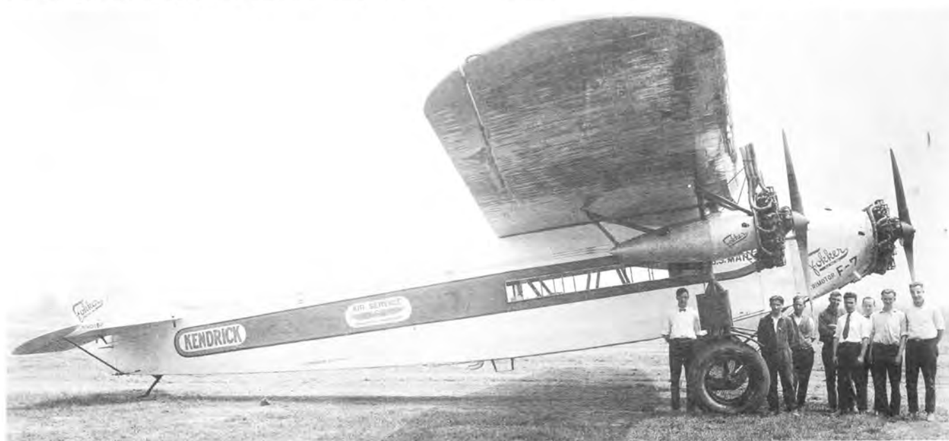
The first two F-VII Trimotors of the Philadelphia Rapid Transit Airline, from Philadelphia to Washington, were named KENDRICK and WILBUR for the mayors of the two cities. KENDRICK carries designation FOKKER TRIMOTOR F-7, while WILBUR used Roman instead of Arabic numerals on nose and tail. Lettering on both, above lower longeron between wing and tail, says: MADE BY FOKKER AIRCRAFT CORP. HASBROUCK HEIGHTS N.J. This in mid-1926 when the company was still known as Atlantic, yet the much later Universal C/N 422 (p 259) was labeled Atlantic. (Am.Fokker from NAA)
