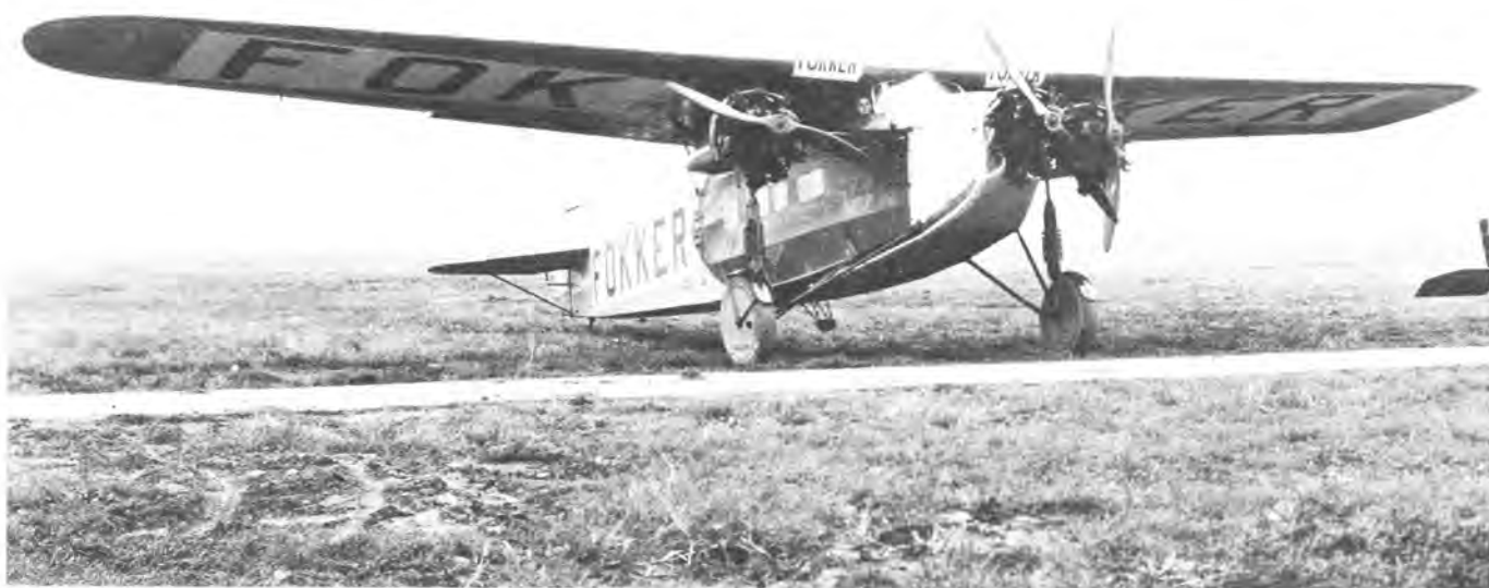
The first Fokker Trimotor under test at McCook Field following the Ford Reliability Tour of 1925. Placement of the markings show the prototype carried standard KLM colors when brought to the U. S. Fokker put his name in the white rectangles used for the European registration. Lettering under cockpit gives designation FOKKER F-VII. Name FOKKER AIRCRAFT CORPORATION appears beneath windows, and letters FAC appear in a winged shield emblem that was the regular KLM emblem but with the Royal crown painted out. (USAF Photo 22381 AC)
