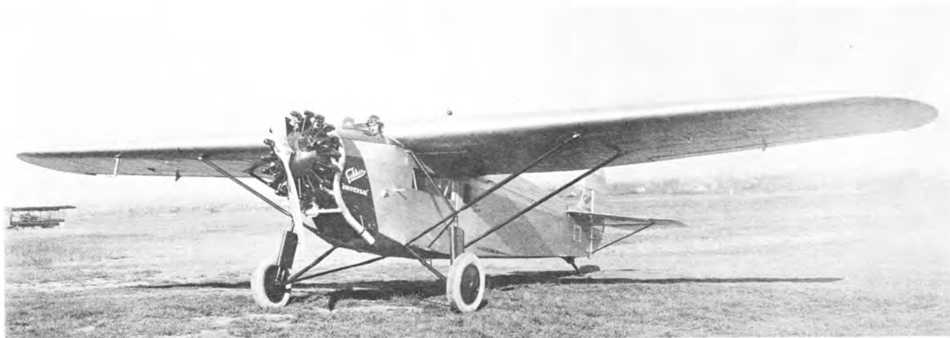
1927-28 production version of the Universal with 220 hp Wright J-5 engine. In spite of Fokker trademarks, lettering above lower longeron behind cabin reads: MADE BY ATLANTIC AIRCRAFT CORP. HASBROUCK HEIGHTS N. J. USA. Although the plane has no registration number painted on, the C/N painted above lower longeron between forward struts as SERIAL #422 (an unusual practice) identifies the plane as an export model for England, G-EBUT. (American Fokker 615)
