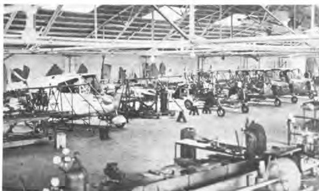
Six Waterman Arrowbiles while under construction. (Matt)
