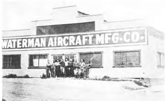
Early employees stand before the Waterman Aircraft Manufacturing Company building, Santa Monica. (Paul Matt)
