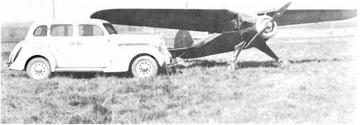
Plymoucoupe with 1935 Plymouth Sedan from which engine, components and trim were taken for use in the airplane.
