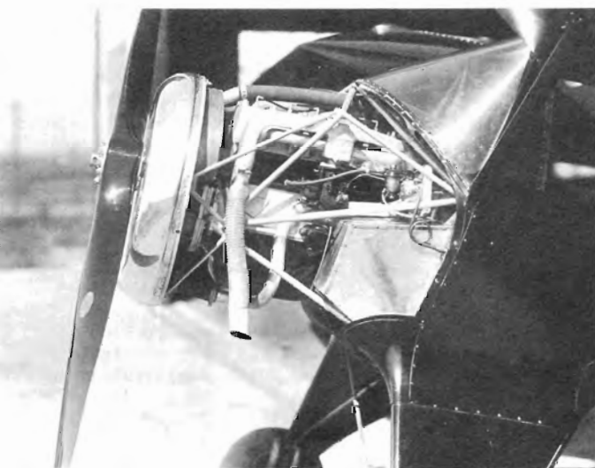
Two photos showing both sides of the Plymouth engine installation in the Plymoucoupe.
