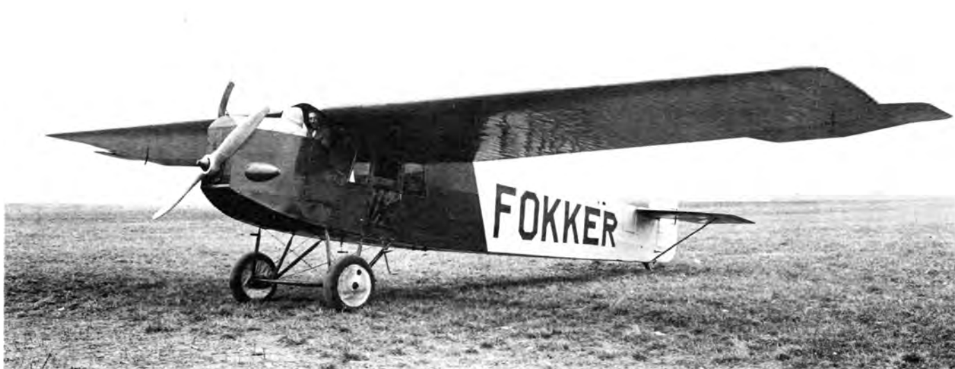
Fokker F-III with the pilot's cockpit offset to the left. Bert Acosta is seated in cockpit. (American Fokker 309)
