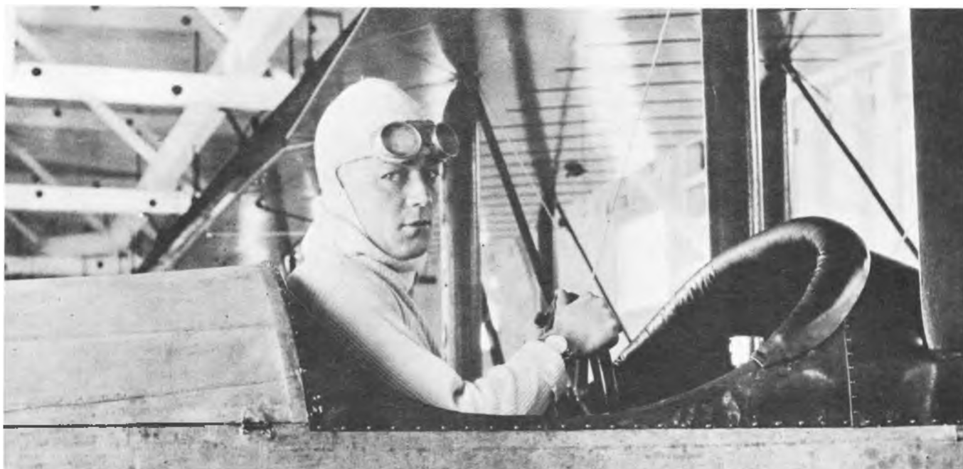
Knox Martin at the B and W controls inside Lake Union Hangar. (Photo - Harold Jensen via The Boeing Co. P32376)
