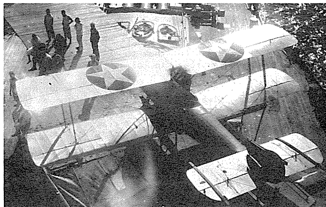
The 1½ Strutter, after being lowered to turret platform, is put into position with tail skid placed in trough.
