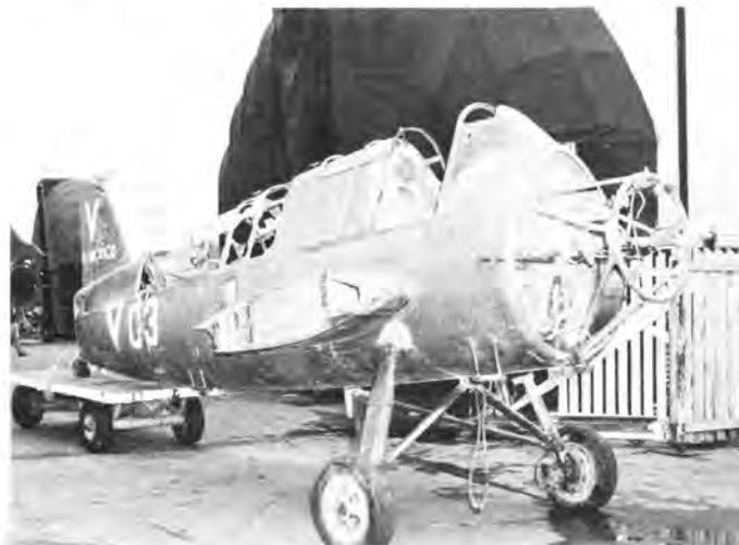
The USS Alabama Battleship Commission Kingfisher as it was when returned from Mexico to Brookley AFB. The tail assembly, wings, cowling, cowl flaps and control surfaces were intact and in good condition. (Edington)
