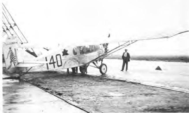
On October 9-10, 1930, the "Columbia" spanned the Atlantic Ocean for the second time. (Photo - F. Ezquerro)
