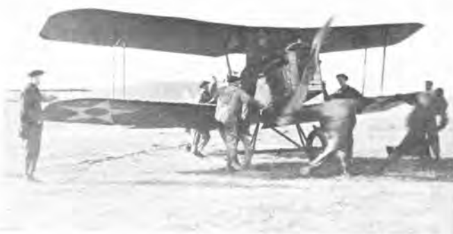
Starting the engine of an SE-5 was a teamwork job although the "team" attending this one is considerably larger than normal. (Photo - Olmsted Collection)
