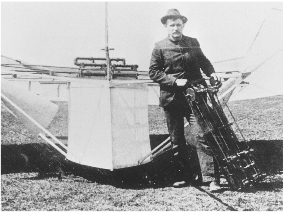
Close-up view of the front of No. 21 with Whitehead holding the 10-hp ground-wheel drive assembly.
