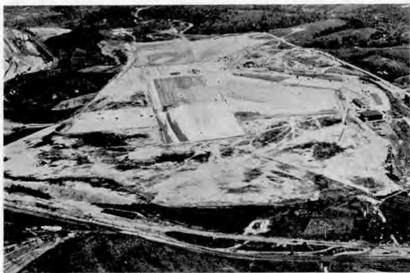
WORK ON NEW PITTSBURGH PORT
