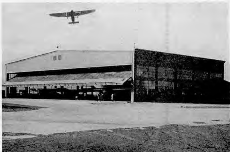
NEW DENVER PORT HANGAR
