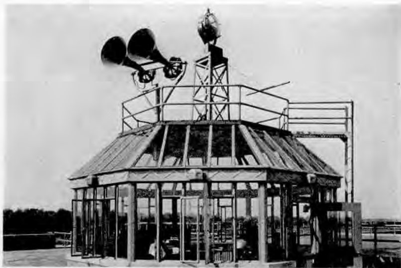
TRAFFIC CONTROL TOWER
