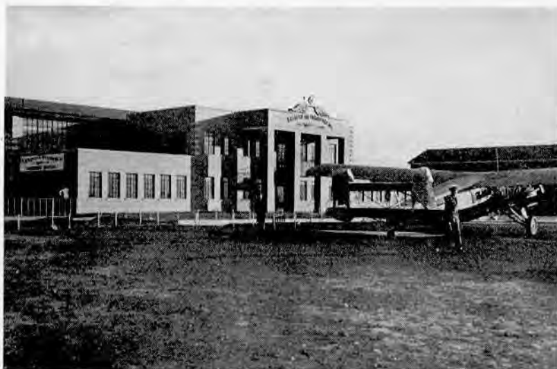
NEW STATION AT NEWARK
