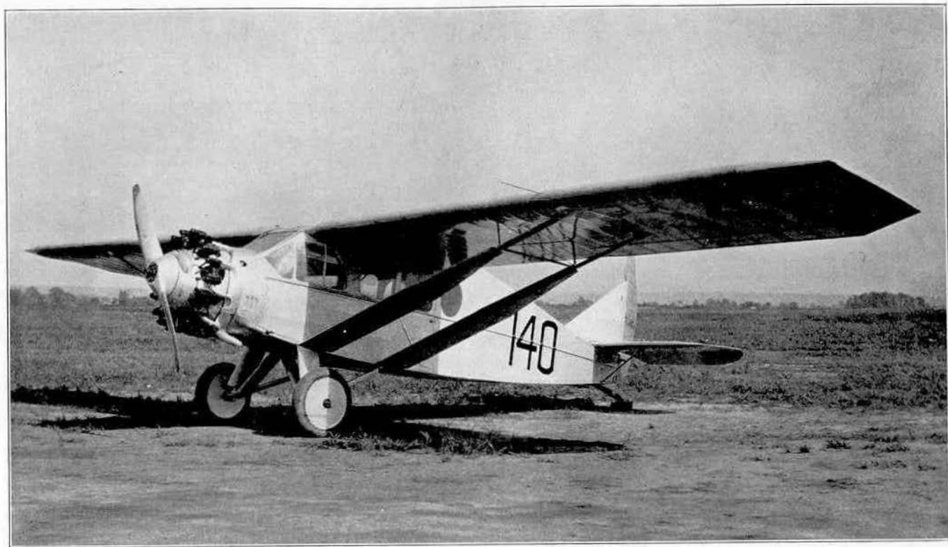
Wright-Bellanca flown by Chamberlin to Germany. Engine, Wright "Whirlwind."
