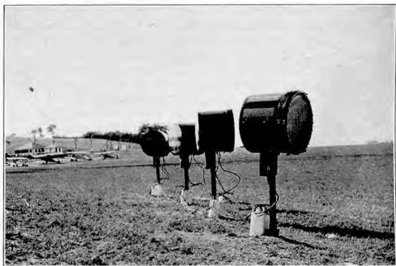
Grouped System of Westinghouse Airport Floodlight Projectors, Bettis Field.
