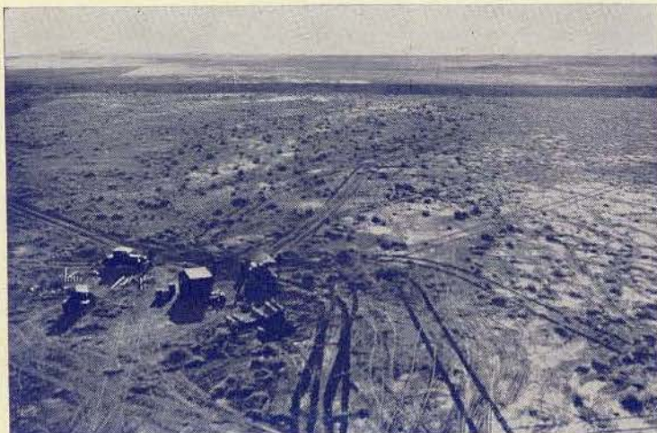
The group of men in the center of the photograph is the crew of engineers and workmen preparing the airport at Waynoka, Okla., for the use of the multimotored TAT planes. The wide runway is shown in the background.
