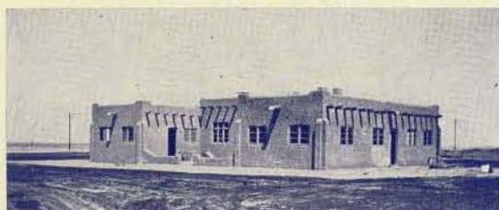
This passenger station at Albuquerque, N. M., is done in the old Spanish style of architecture familiar to the region. It is one story of tile and stucco. In one wing are the waiting rooms, newstands and restrooms. The other wing is occupied by TAT offices.
