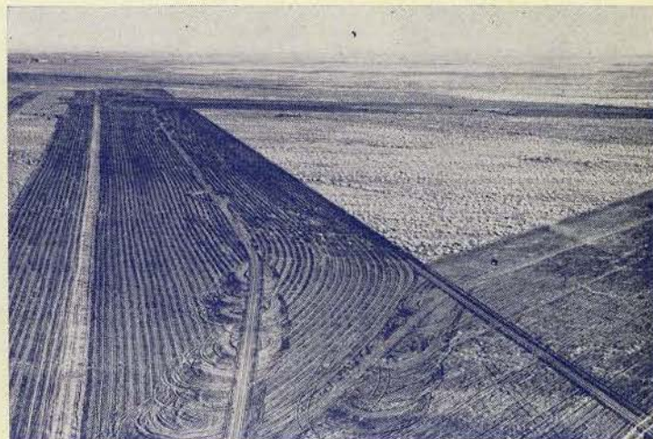
Each airport is furrowed repeatedly and the soil subjected to an intensive oil treatment which makes the runways water-proof and removes the dust annoyance. The photograph is of the furrowed runways at Kingman, Ariz.
