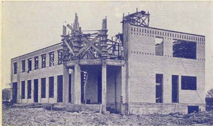
(Left) The municipal passenger station at Port Columbus, two stories high and of light faced brick, will have a complete waiting room, restaurant, newstands, ticket offices and on the second floor, the TAT field office, pilots' rest-rooms and a tower for the field director. It will be completed before July 1.
