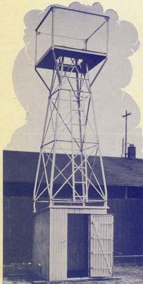
Beacon lights placed at regular intervals along the TAT airway, and at airports, for the guidance of pilots at night, will be erected on towers such as this one.
