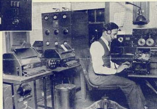
Interior views of radio and tele-type installations. The upper photograph is of the radio control panels and the receiver. The narrow tape which the operator holds in his hands has just come from a tele-type machine.
