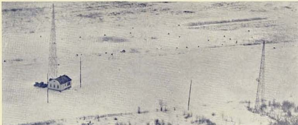
An aerial view of radio "shack" and towers being installed at all TAT airports. The towers each are 128 feet tall.
