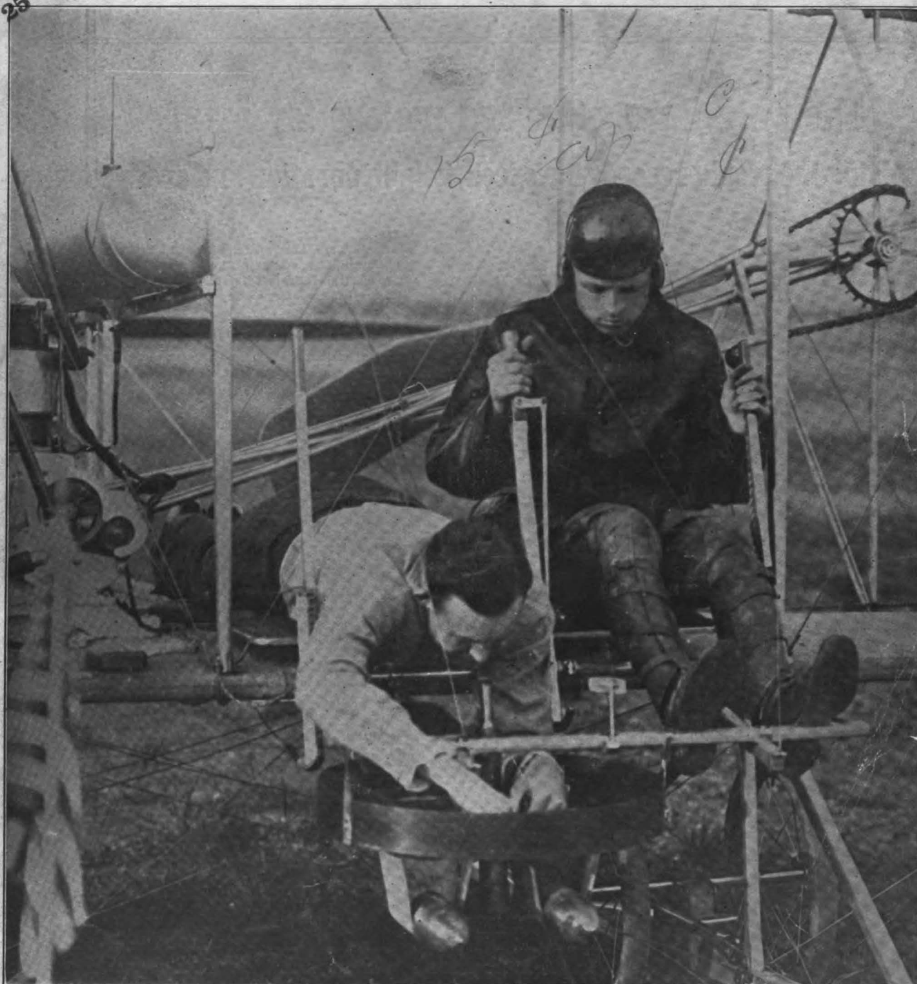
LIEUT. SCOTT ADJUSTING HIS BOMB DROPPING DEVICE BEFORE STARTING ON A TEST FLIGHT IN AN ARMY BIPLANE, WITH LIEUT. MILLING AS PILOT
