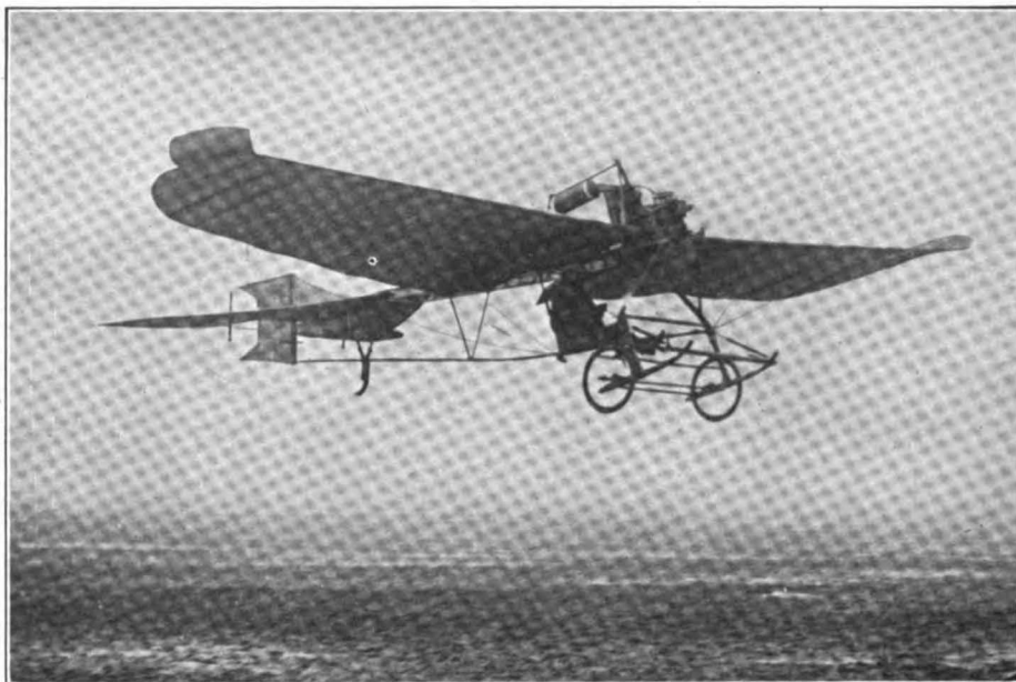
THE VINET MONOPLANE IN FLIGHT. THIS MACHINE IS OF AN IMPROVED DEMOISELLE TYPE AND HAS BEEN QUITE SUCCESSFUL IN RECENT TRIALS. IT SHOULD BE A VERY EASY MACHINE TO CONSTRUCT.
